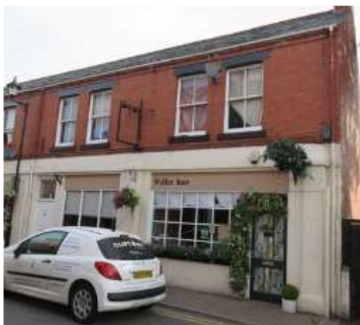
Cellar Door Exterior
