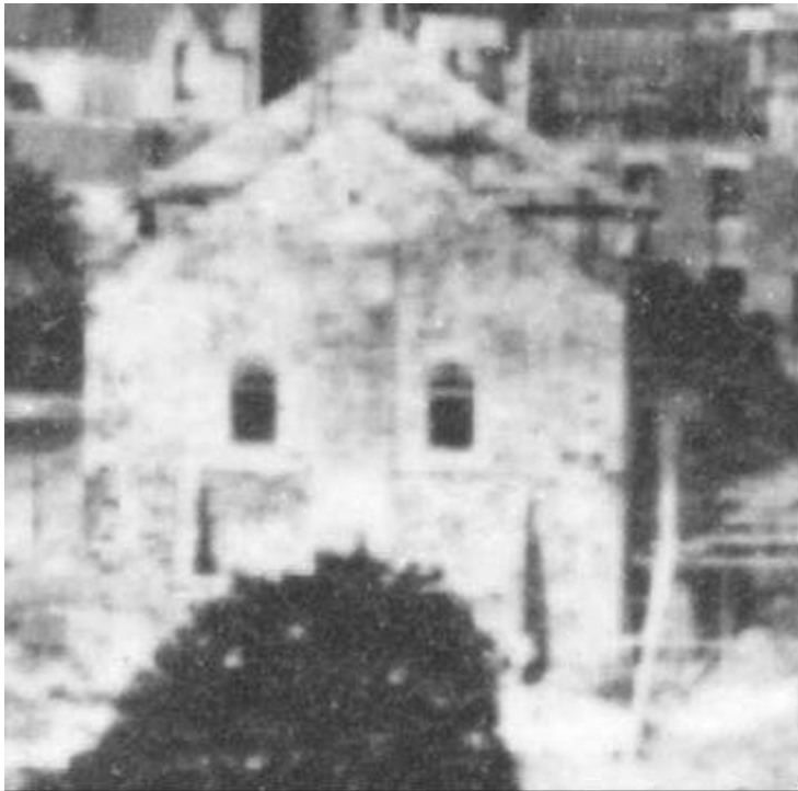
1860 (from rear during construction)
