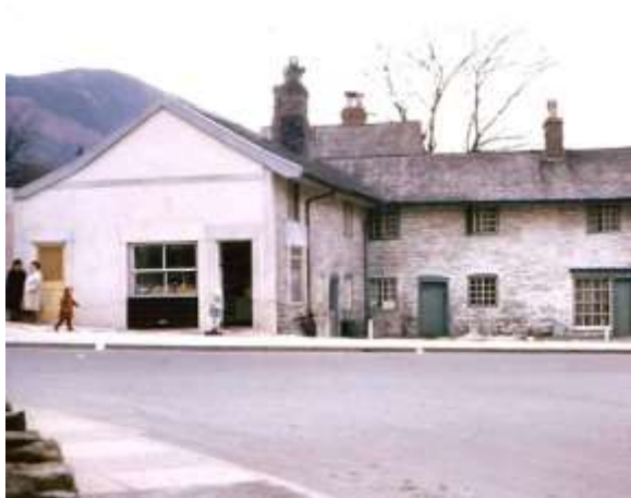
Immediately after bridge widening
