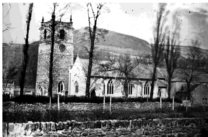
St Collen's Church around 1880. The relatively new south aisle and the chancel at the east end can be seen.
