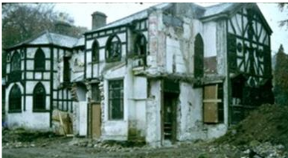
The demolition in progress in 1963.
