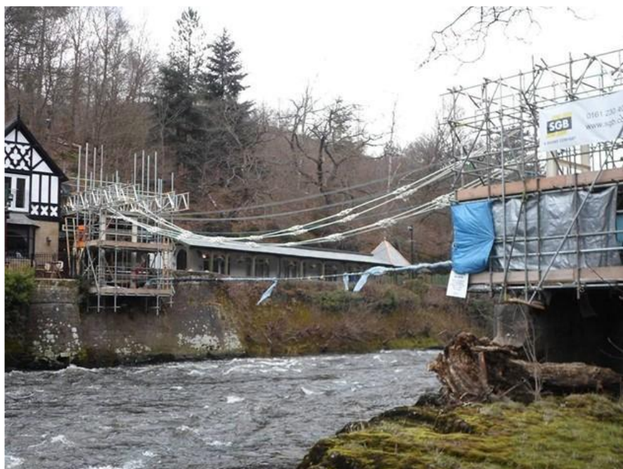
The bridge being dismantled
