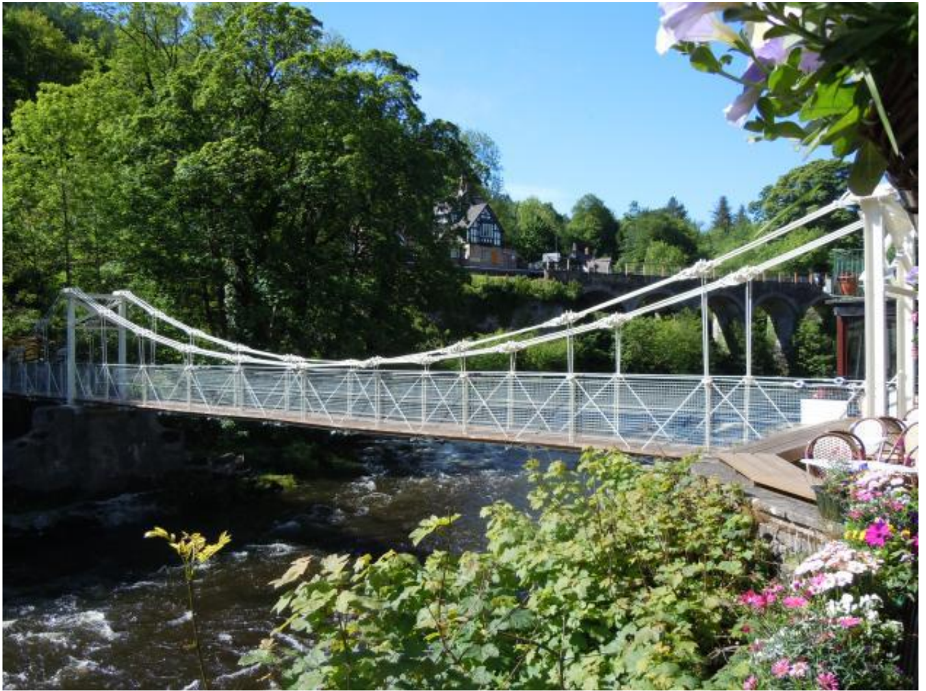
The Chainbridge after restoration
